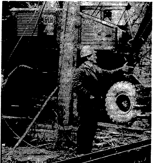
John Matthews, "The Old Boom Picker" from Buffalo, working for the Ford Pile Driving Co. of North Tonawanda, gives the signal for "boom up" while the crew were driving piles for the foundation of the new Second Street Bridge now under construction. (News Photo)
