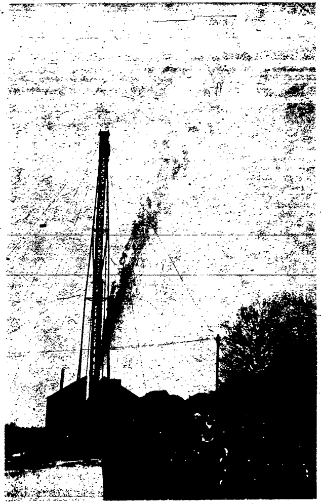
The oil well on the Linford Potter Farm seconds after it was shot. Photo by Wittie
