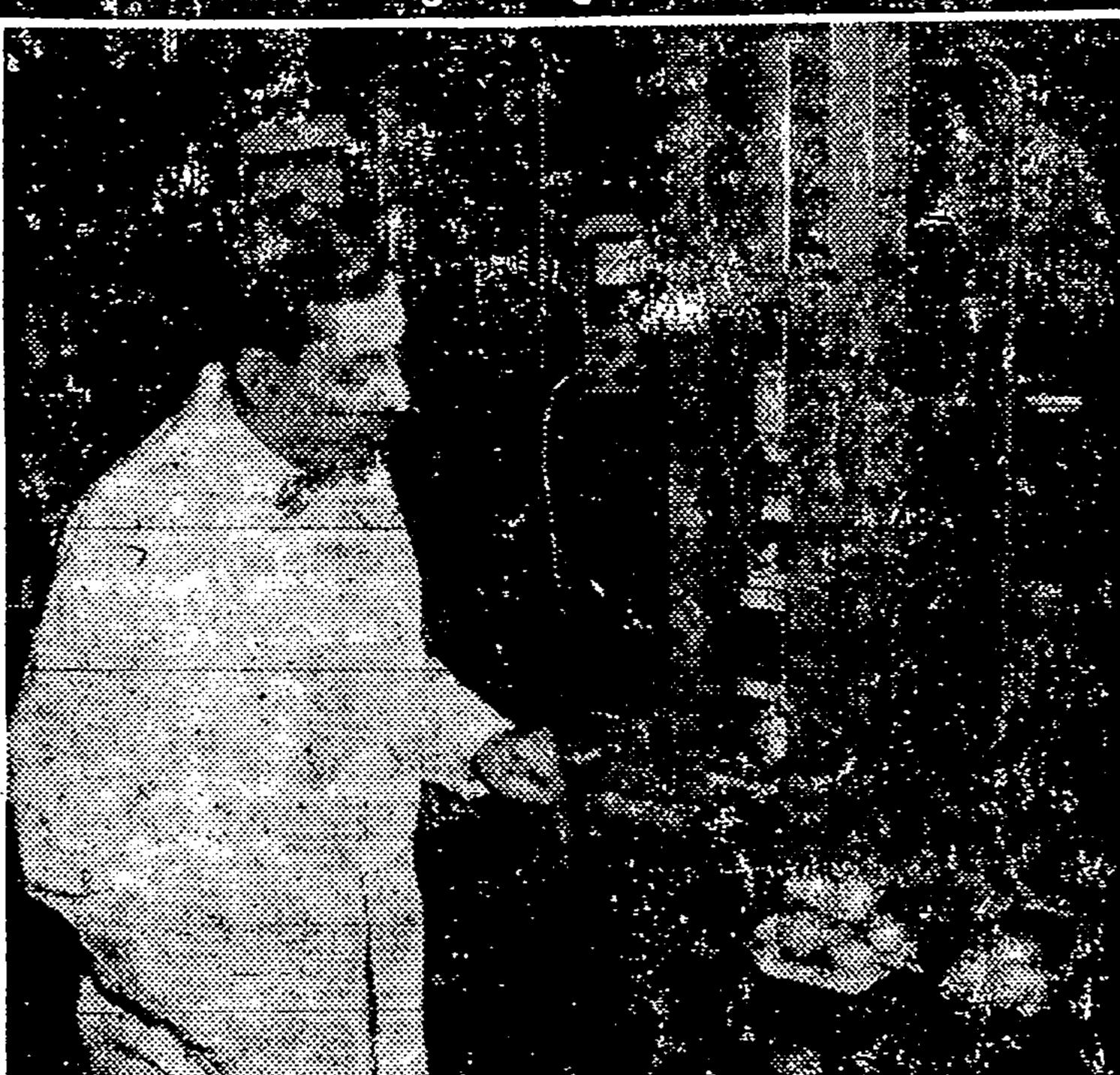
PUTTING ON THE SQUEEZE—How much pressure can an onion take before it breaks? It's an important problem in bulk storage where onions at the bottom of 10,000 to 40,000 bushels sometimes become misshapen and unmarketable. Here, Prof. F. M. Isenberg of Cornell is testing firmness and hardness in different varieties. Altegether, 15 varieties will be tested both in the lab and un actual storages. Bulk storages reduce producer costs, and if widely
