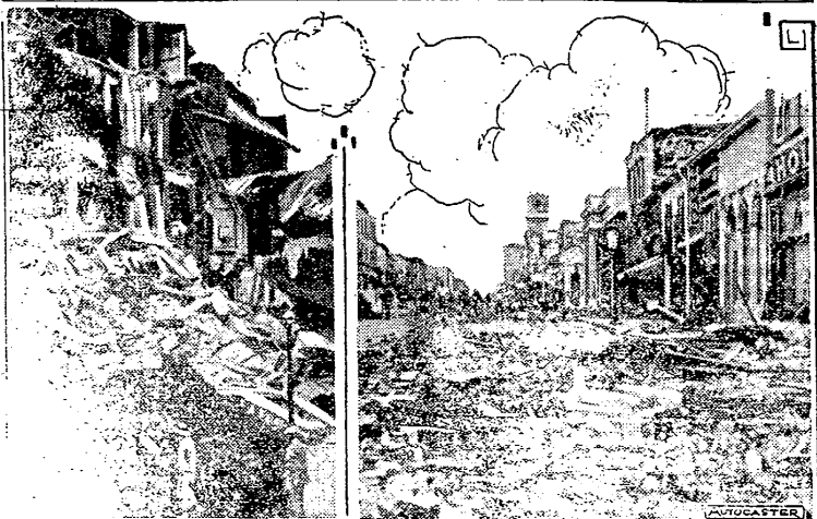
These are two remarkable pictures, sent by telegraph, of the ruin in Santa Barbara, Calif., caused by the quake. At the left, the photo shows the ruins of the famous Arlington Hotel, almost completely destroyed. At the right—a view of State Street—principal business thoroughfare—as it looked one week after the quake.
